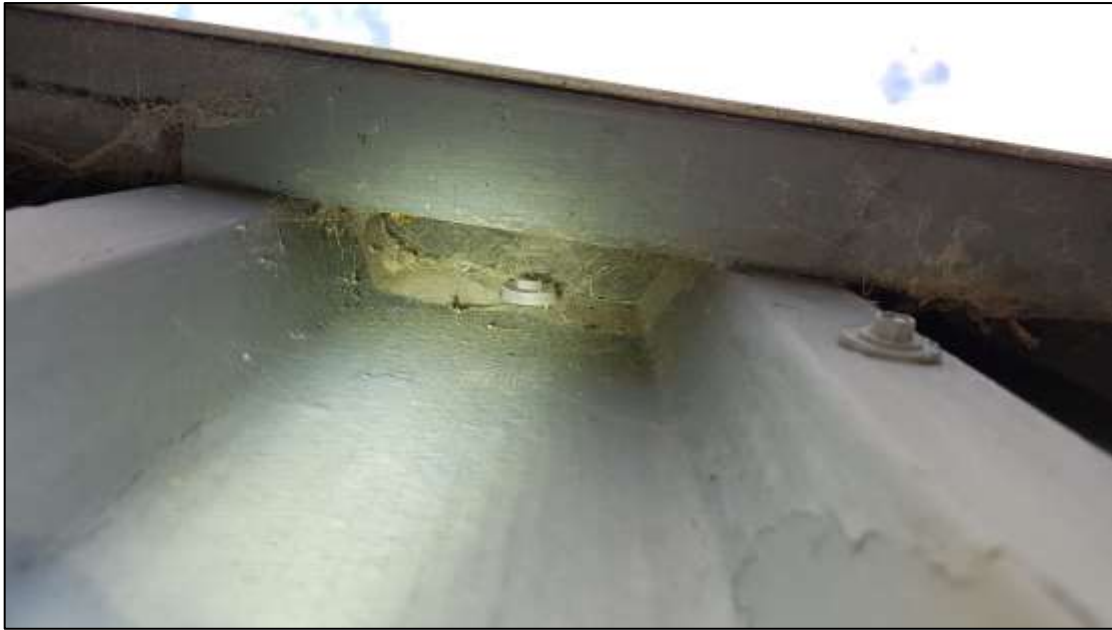
Plate 14: All gaps in the eaves were sealed up with no potentially suitable areas of entry.
