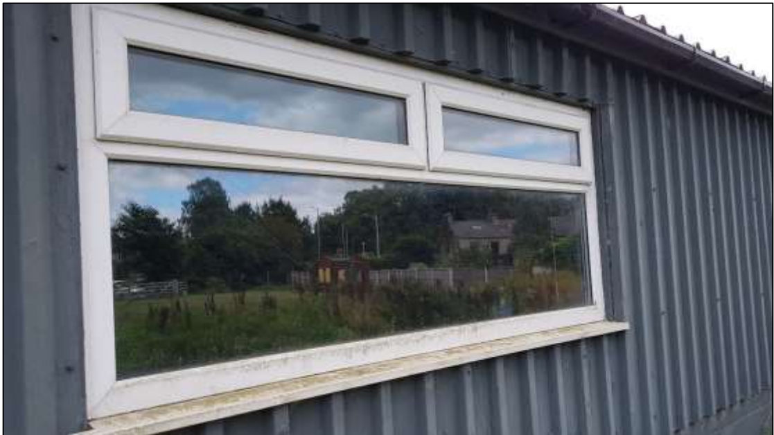
Plate 13: All windows and doors were fully sealed around the building.
